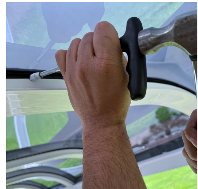
Use a round edged piece of wood or plastic to hit or push the rubber into the groove.
